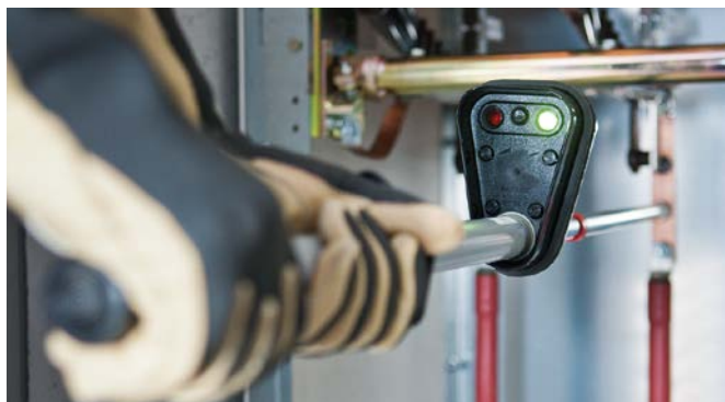
PHE voltage detector with visual indication.
