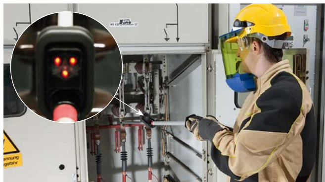
PHG II voltage detector used in a type-tested switchgear installation.
