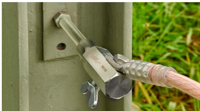
Fixed earthing point with ring groove and earth bushing.
