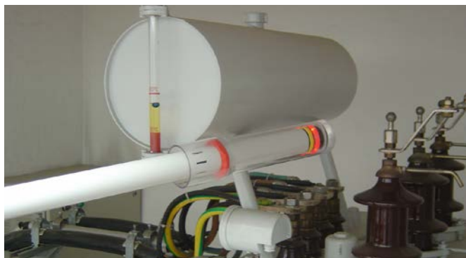
HSA 205 high-voltage indicator with insulating cap used on a switchgear installation.
