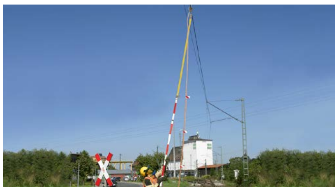
Attaching a railway earthing device.
