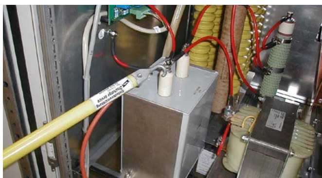
Single-pole device for discharging static charges.
